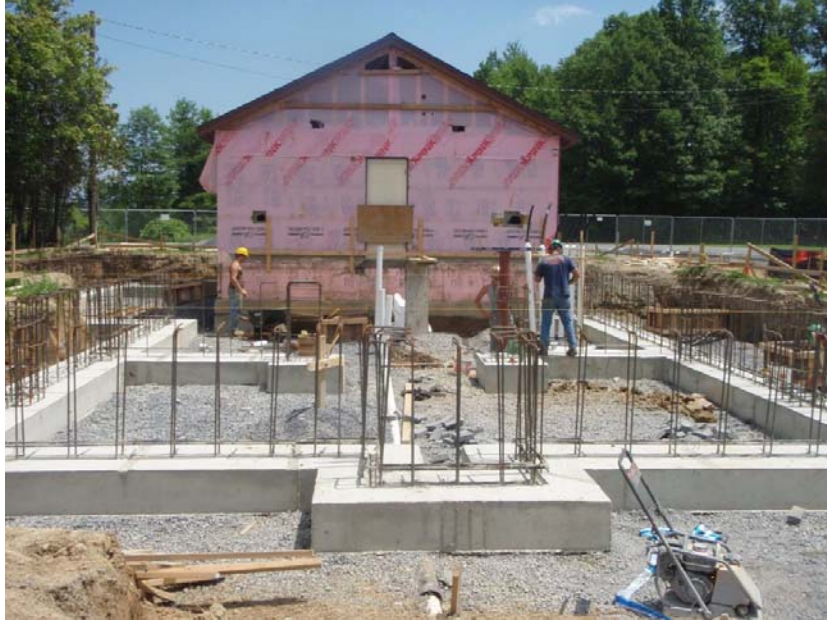
The concrete foundation walls have been formed and poured.
