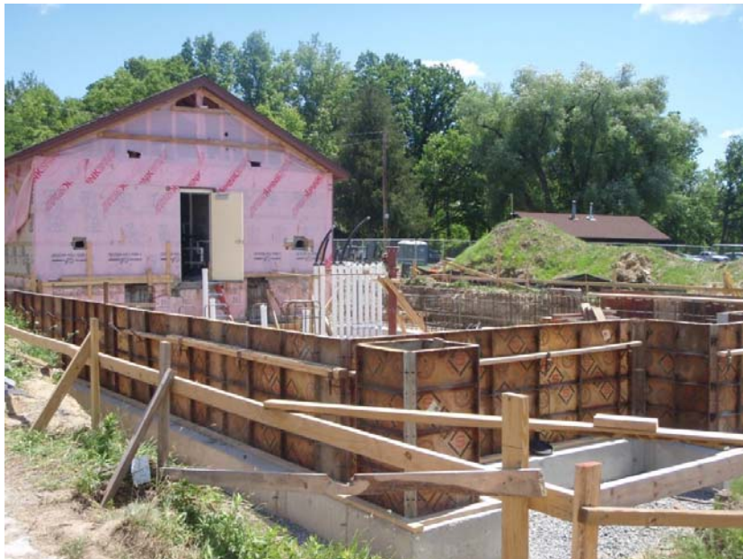
The concrete foundation walls have been formed and poured.
